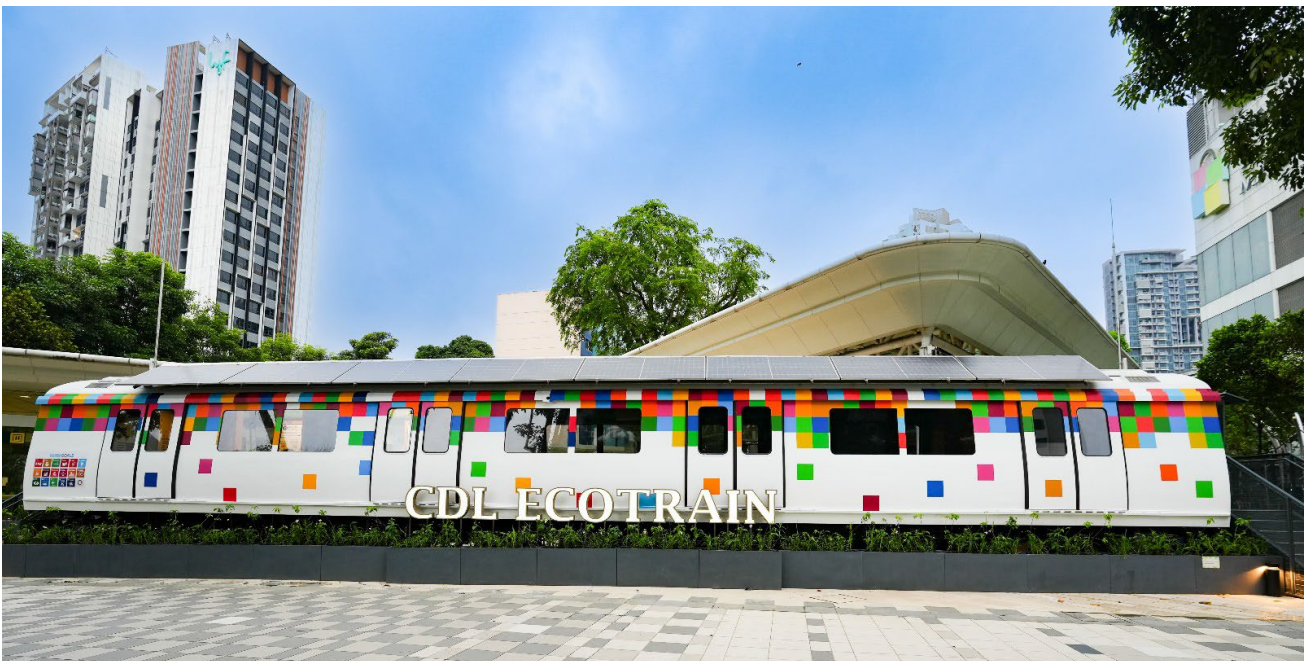
The decommissioned SMRT train cabin has been repurposed into a zero-energy CDL EcoTrain. The cabin is designed with colours and messages inspired by the 17 United Nations Sustainable Development Goals (UN SDGs).
